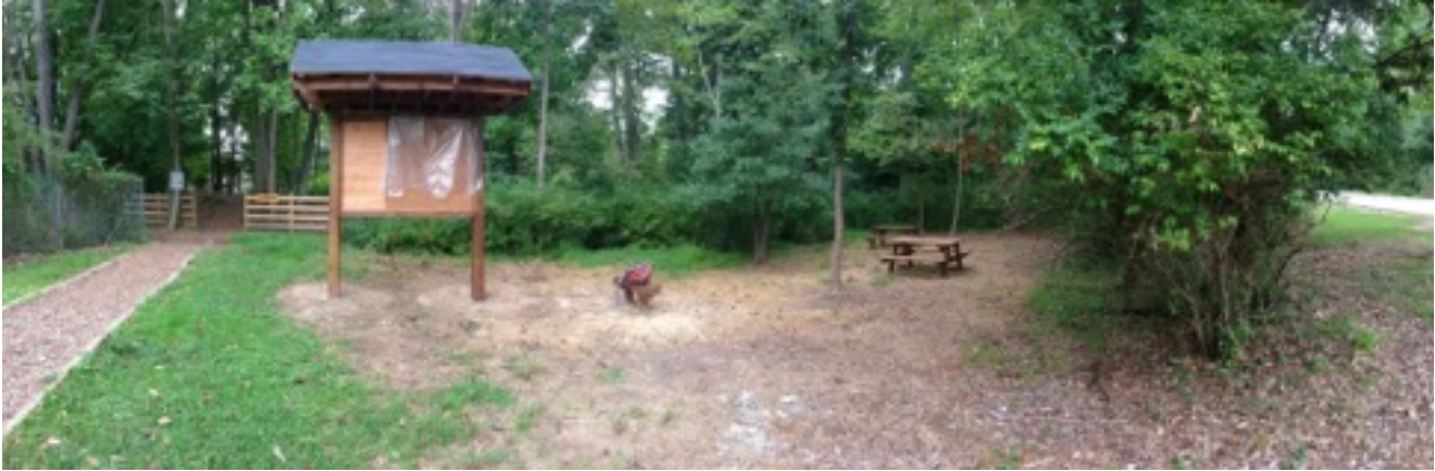
Body and trailhead were combined and pulled up and placed in the pre-dug post holes. Concrete was then used to completely secure the trailhead.
