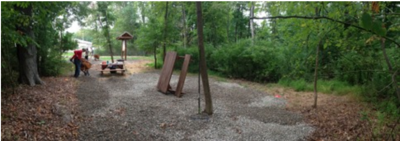
Approximately 2 inches of stone were laid down as a base. This will help with draining and prevent flooding later down the road.
