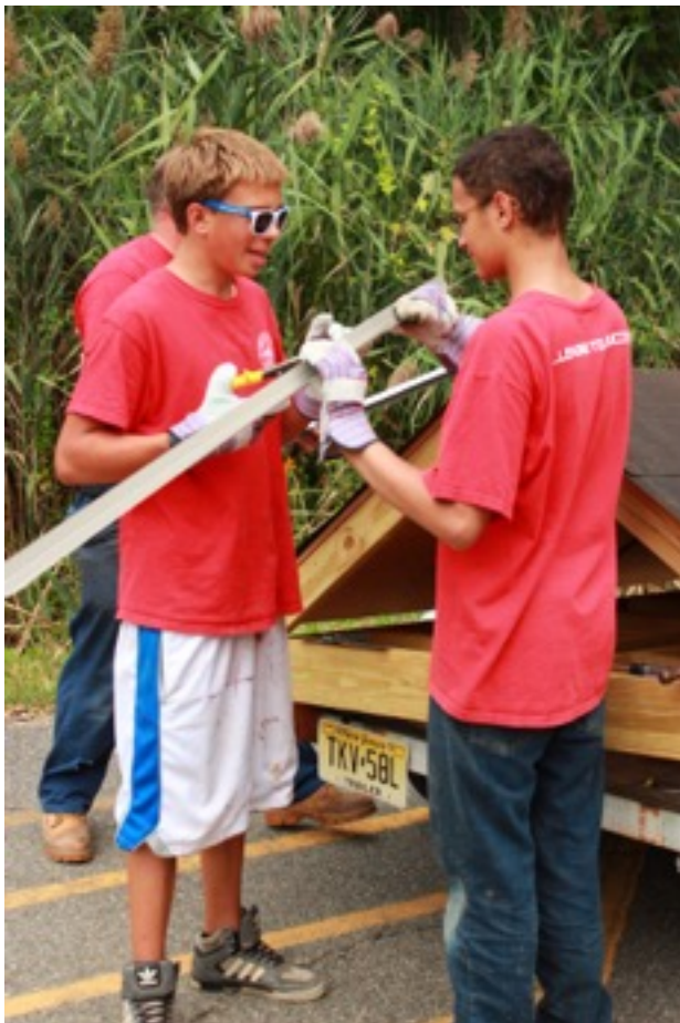
Drip edge was cut using tin-snips. Volunteers are wearing safety gloves to protect them from the sharp edges.
