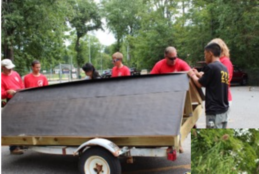
Nailing in the starter strip of shingles that went over the the roofing paper. Eventually the entire roof was covered in shingles.
