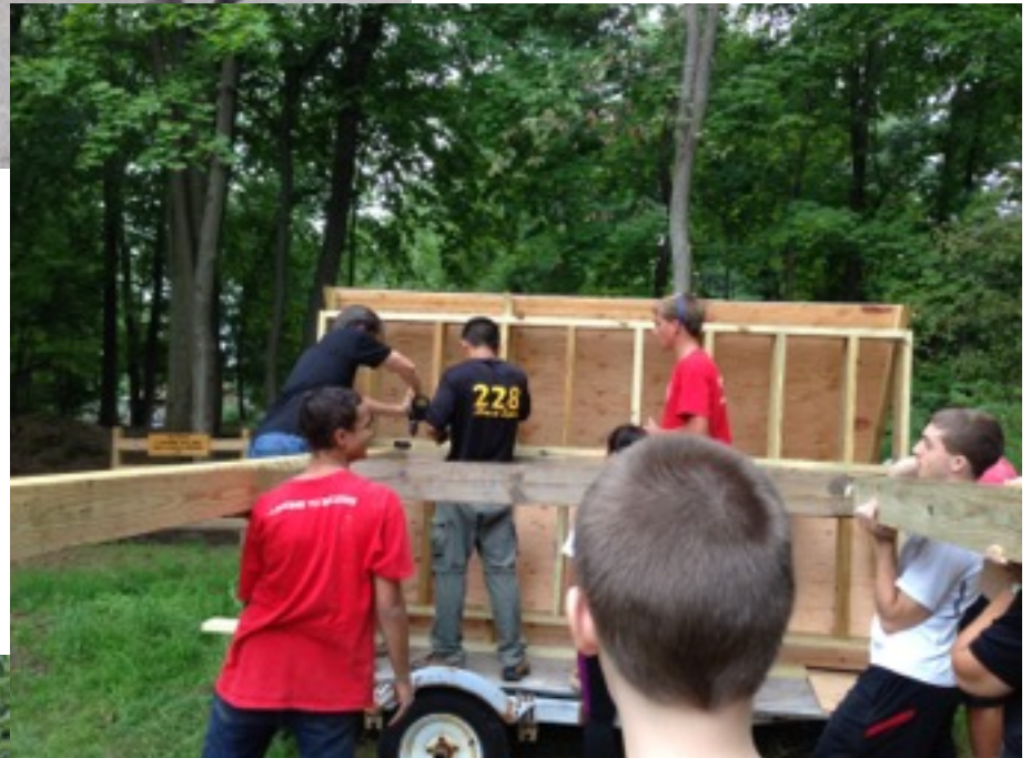
The posts of the trailhead were then positioned over the pre-dug holes.
