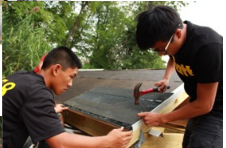
Drip edge was cut using tin-snips. Volunteers are wearing safety gloves to protect them from the sharp edges.
