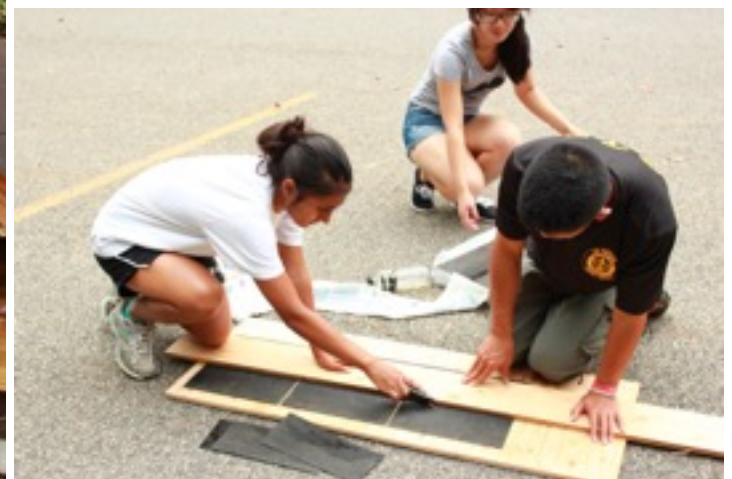
While cutting the shingles, excess plywood was used as a guide to help with the cutting process.
