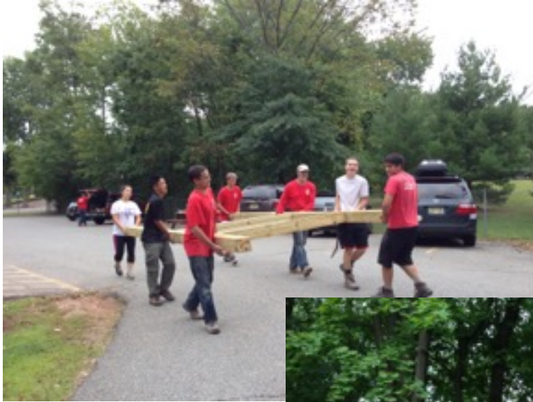
The body of the trailhead was carried into position and then secured with carriage bolts.
