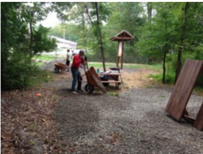
Approximately 2 inches of stone were laid down as a base. This will help with draining and prevent flooding later down the road.
