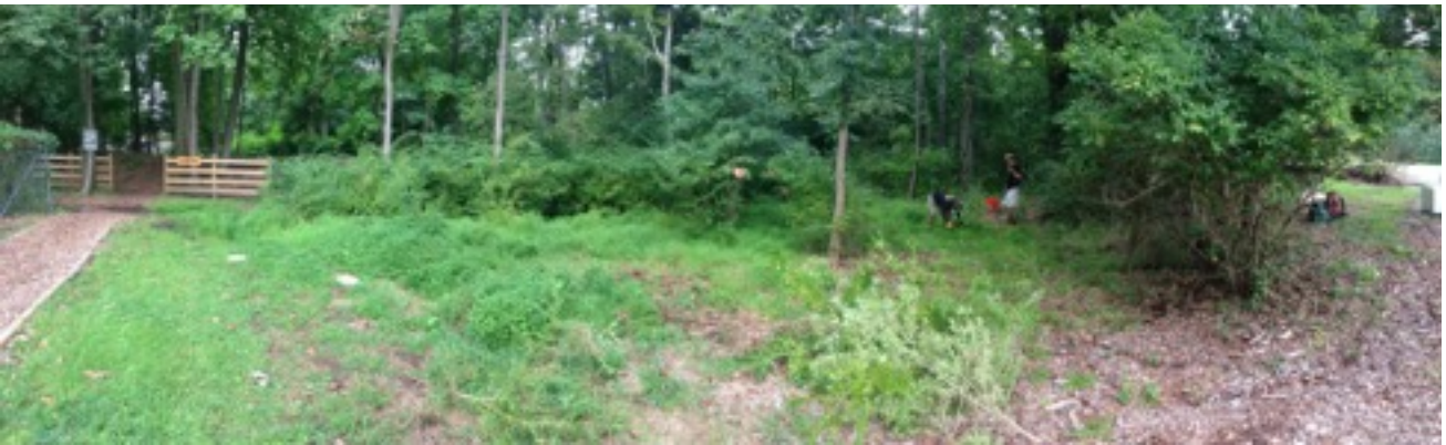
Work at the grotto has begun. Scouts are helping to cut down larger bushes and remove the brush within the set perimeter.
